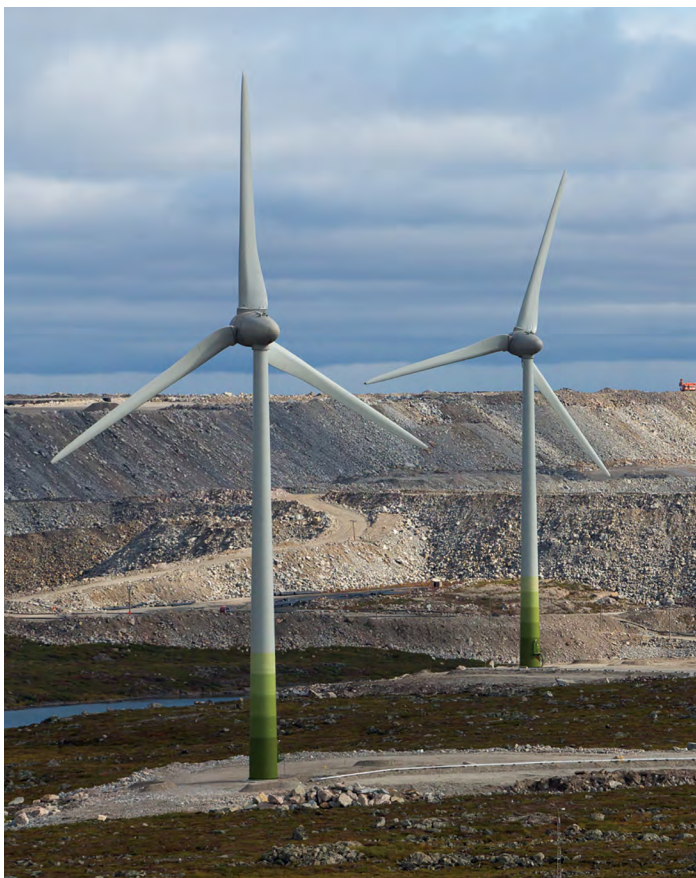
At Diavik diamond mine, Rio Tinto operates one of the largest hybrid wind-diesel power facilities at a remote mine site in the world. The off-grid mine is located on an island in a subarctic lake called Lac de Gras, in Canada's remote Northwest Territories, and since coming on line in 2012 has offset Diavik's diesel use by over 26 million litres and reduced the overall greenhouse gas emissions by 72 thousand tonnes.
