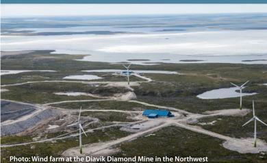
Photo: Wind farm at the Diavik Diamond Mine in the Northwest Territories reduces Diavik's diesel fuel consumption by 5 million litres annually.
