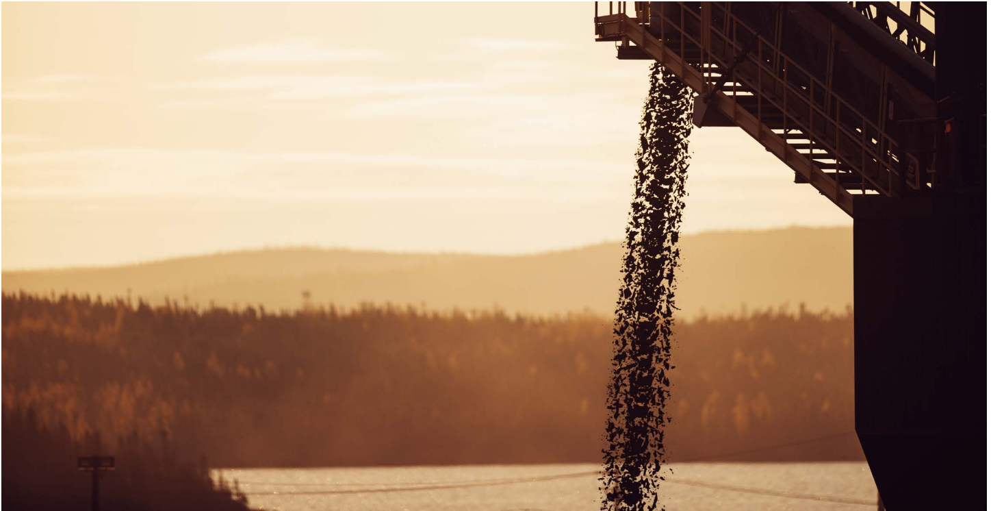
Material going to ground from a concentrator stacker at IOC Operations in Labrador City, Newfoundland and Labrador.
