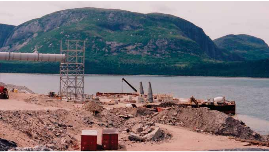
Construction of the Voisey's Bay port facilities
